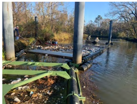
Figure 2.18 Litter Trap Cleaning
